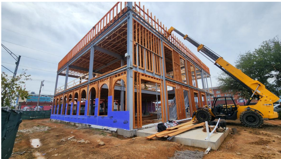
View from Garrison Avenue, August 21, 2026 — steel frame, second-floor deck, roof framing, and the arched storefront arcade that recalls the original Fishback / Adelaide Hall facade.
